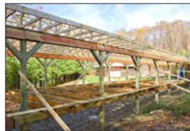
New pole barn construction
